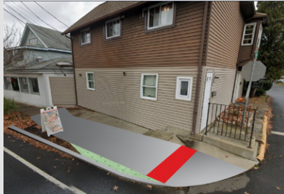
Sidewalk and Drainage Improvements at 132 Shore Drive • Concrete splash block will be installed to reroute water off sidewalk
