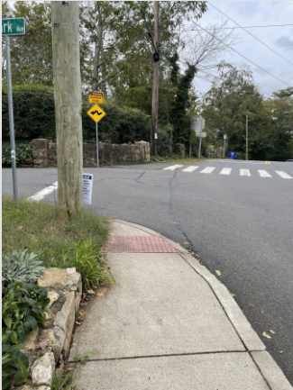
Non-Compliant Crossing Across Clark Avenue
