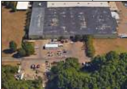
Public Works Facility
