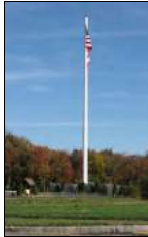
Stealth Monopole As Flagpole
