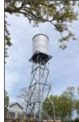
Stealth Installation In Branford
