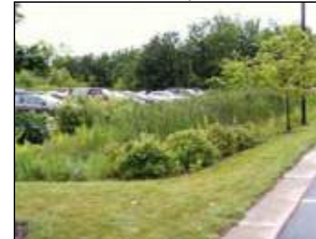
Water Quality Basin
