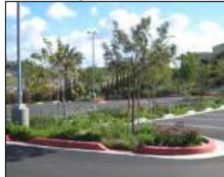
Parking Lot Infiltration Basin
