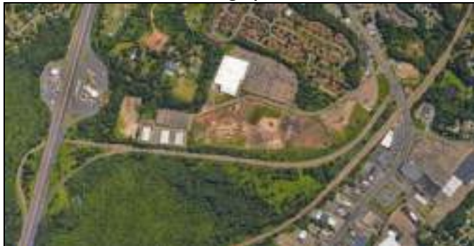
Aerial Photograph Of Exit 53
