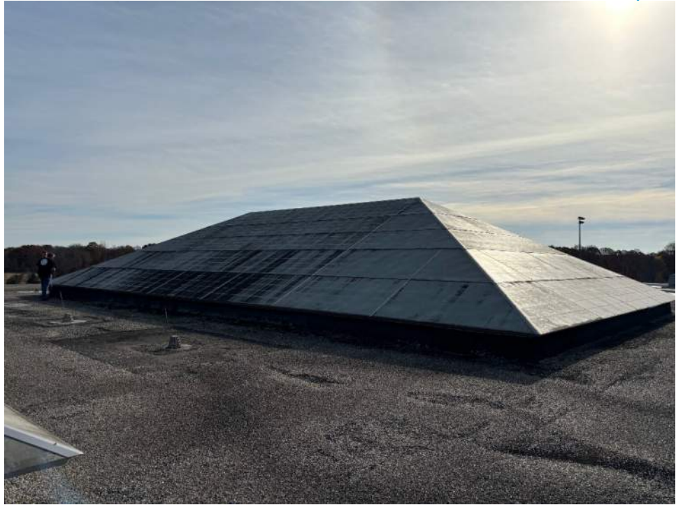
Large skylight at Roof 14
