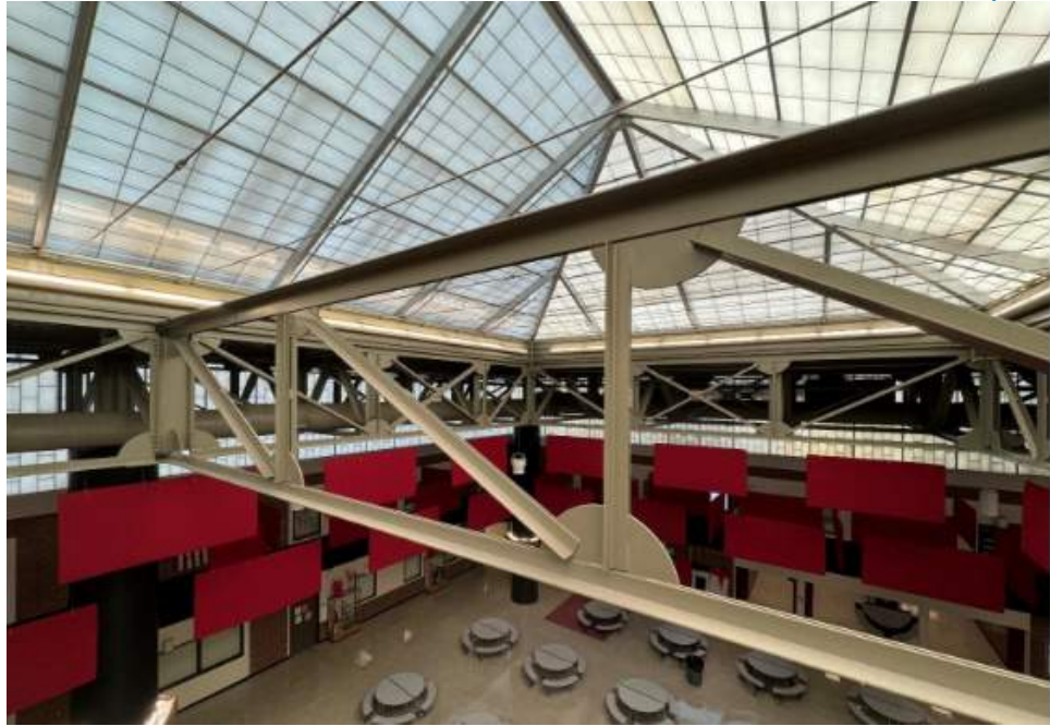
Interior view of skylight. Roof supporting structure.
