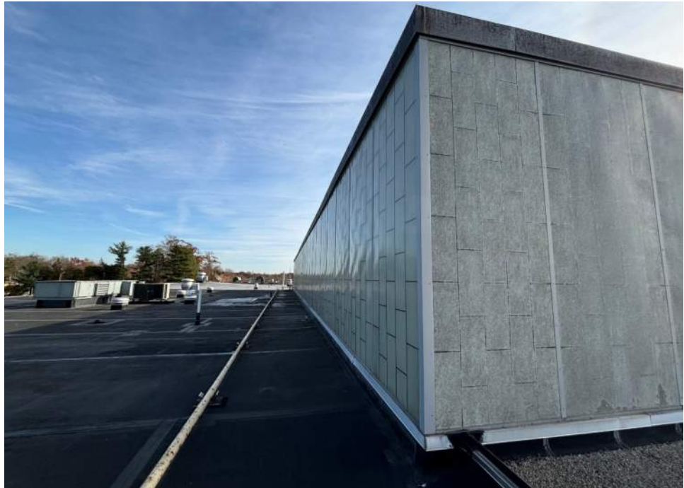
Translucent wall panel at Roof I4 perimeter
