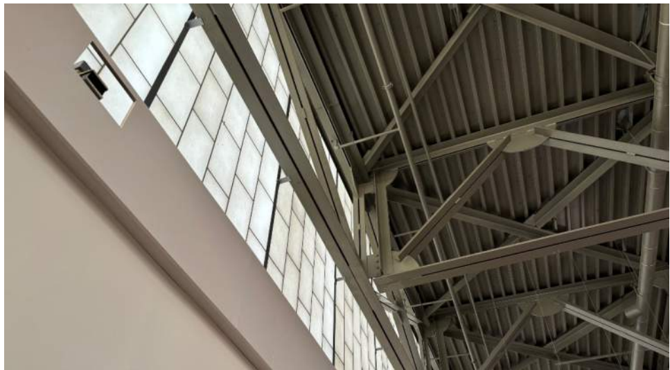
Translucent wall panel at Roof I4 perimeter from the interior
