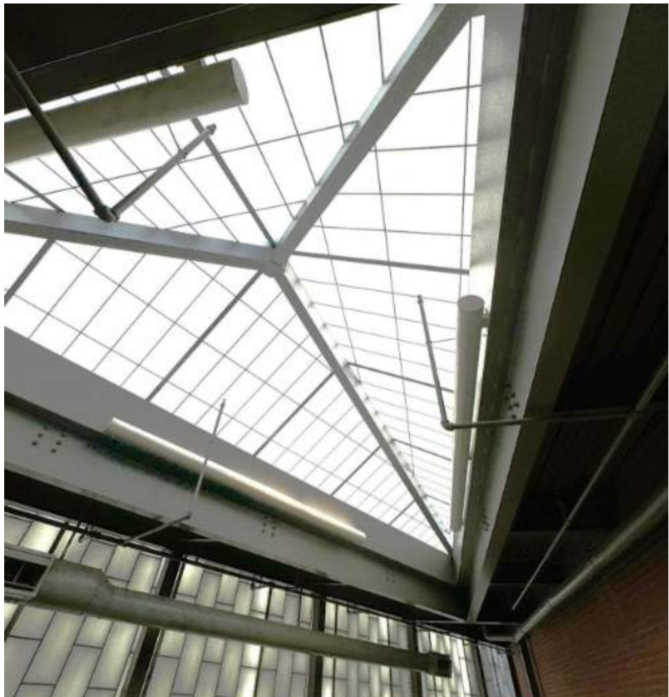
Interior view of Roof 2 skylight and translucent wall panel
