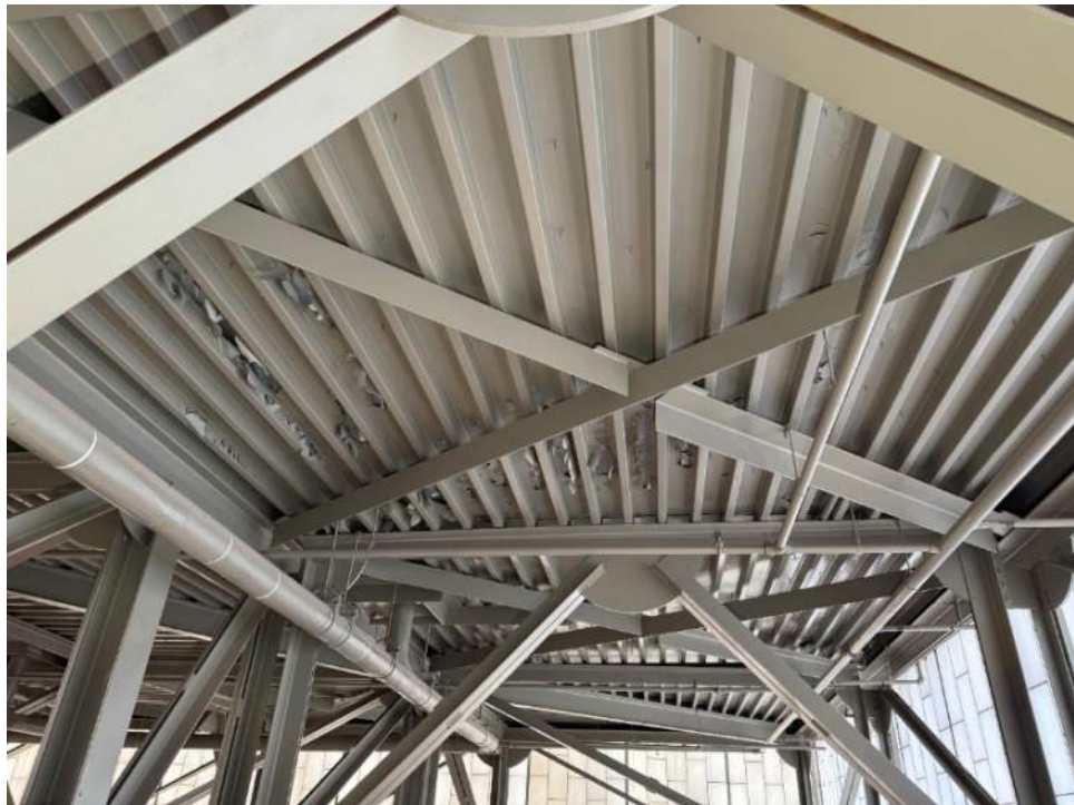
Interior view of roof deck and structure.
