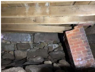
chimney disconnected from stack
