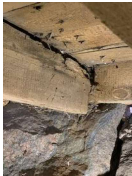
rotting joist
